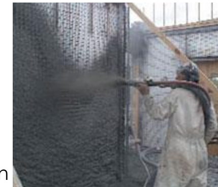
Concrete Spraying
