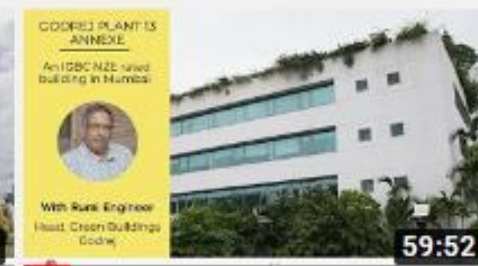
Godrej Plant 13 Annexe -an IGBC NZE Rated Building
