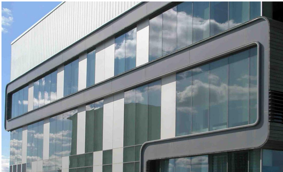
Curtain wall glazing
