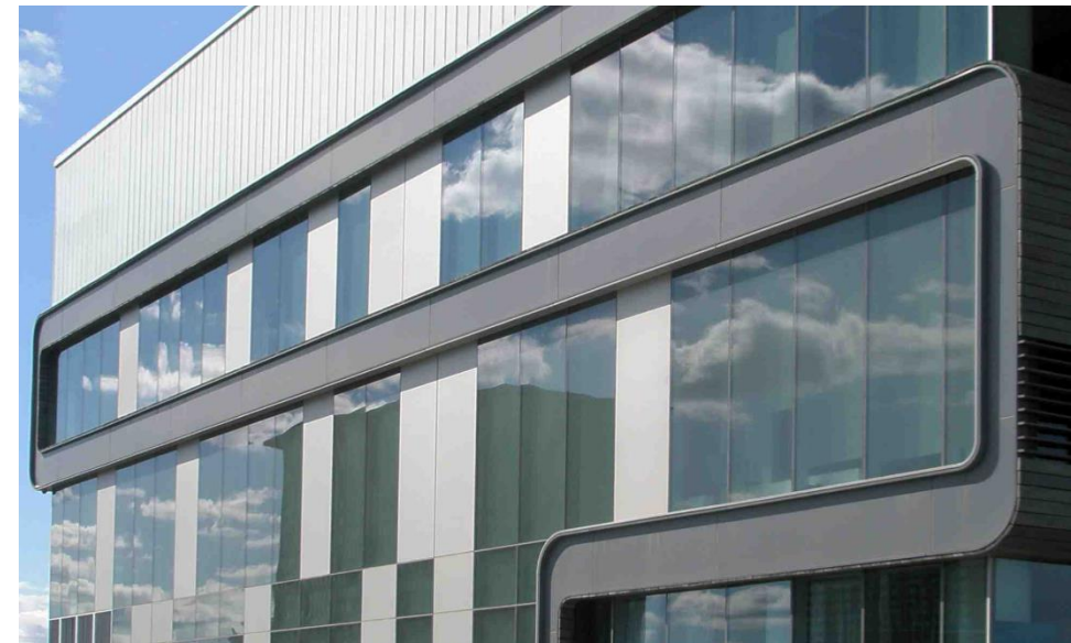
Curtain wall glazing
